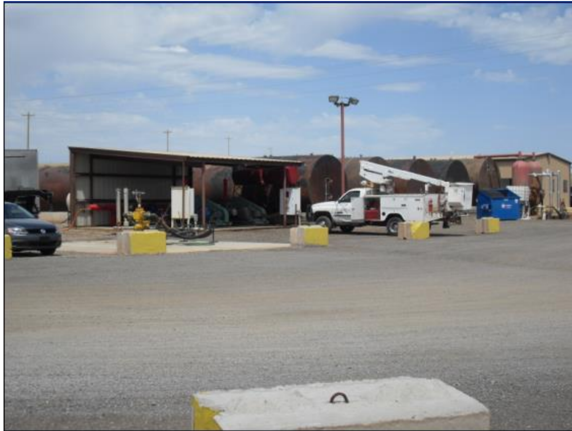
Equipment operating at a waster disposal site - Oklahoma
